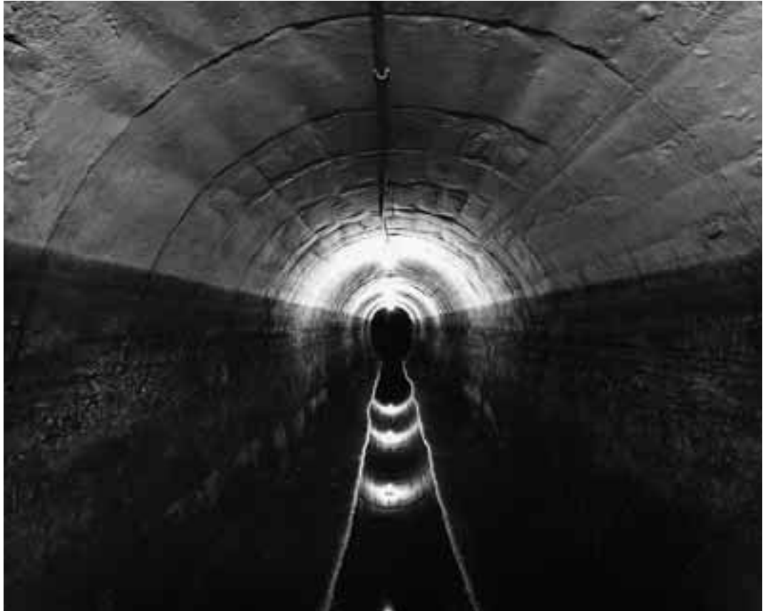
Kuva 1: Old Croton Aqueduct, Ossining, New York, 1997
