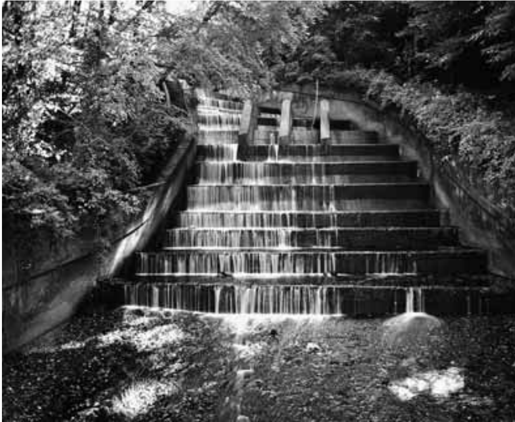
Kuva 2: Spillway, Croton Falls Reservoir, Putnam County, New York, 2000
